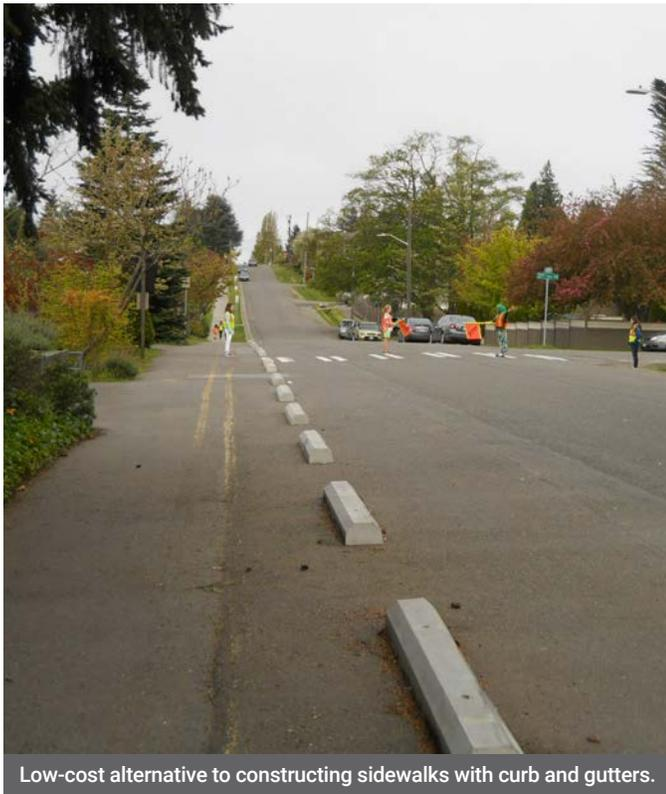
Low-cost alternative to constructing sidewalks with curb and gutters.
