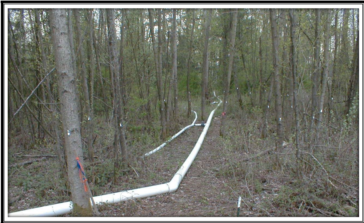
Figure 5.25. Manifold and Branches in a Wooded, Vegetated Spray Field.
