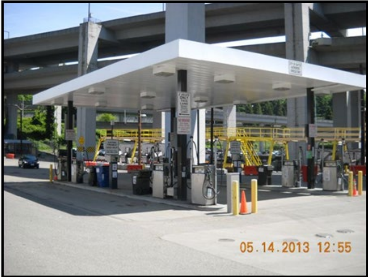
Figure 9.2. Roof at Fueling Island to Prevent Stormwater Run-On.
