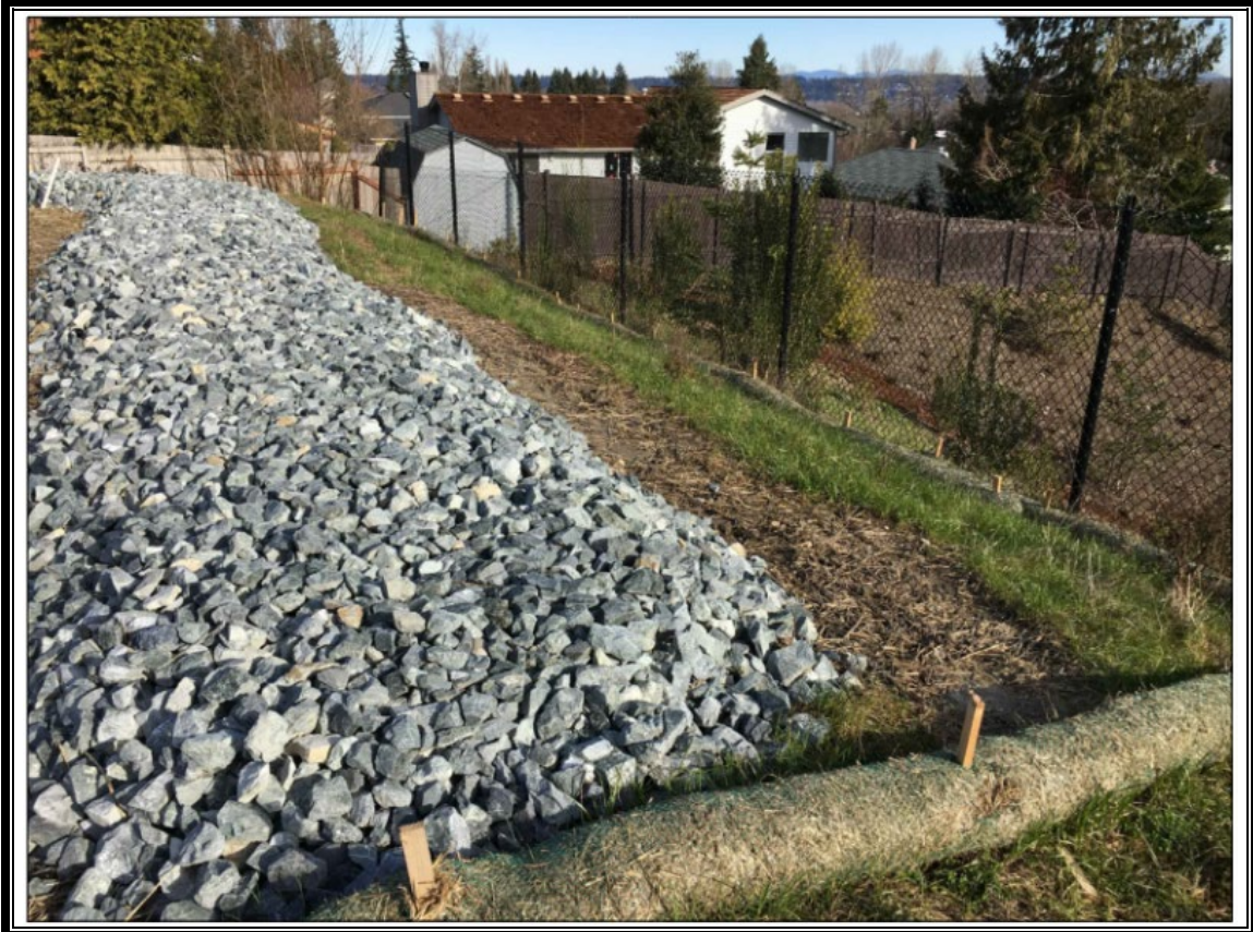
Figure 5.21. Gravel Filter Berm.
