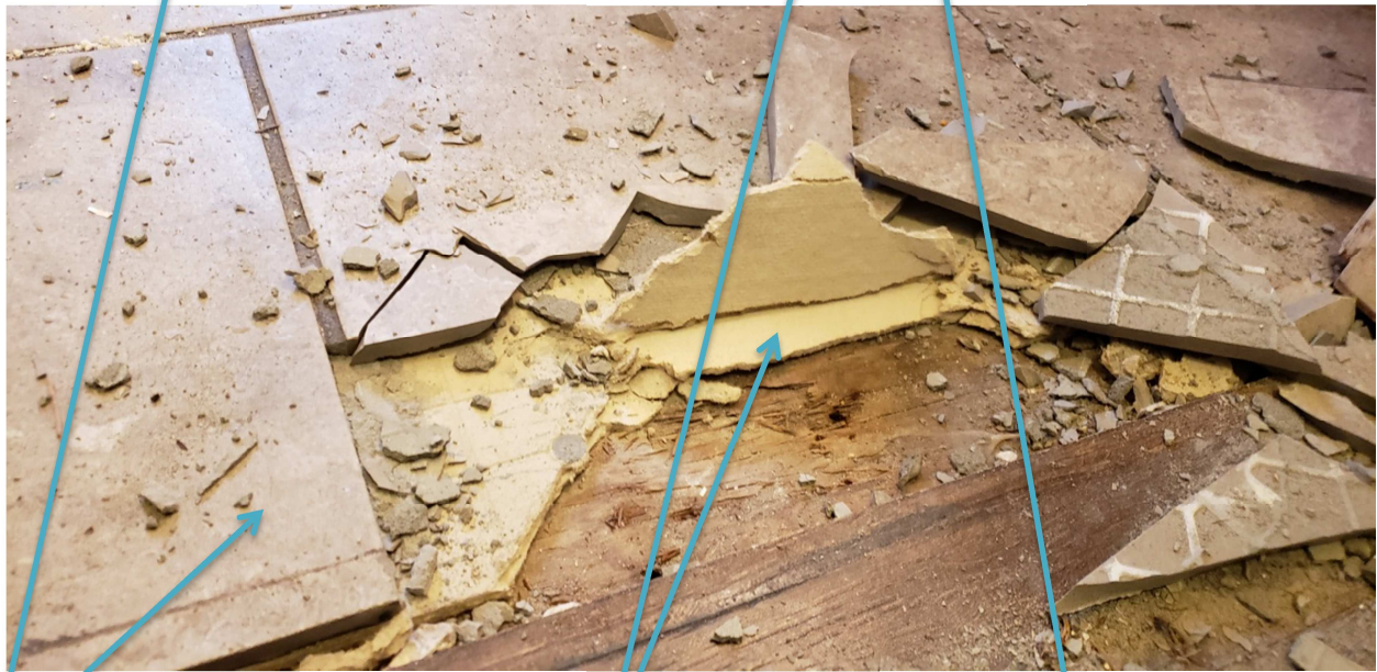
ASB-064- gray tile grout- Non-detect
