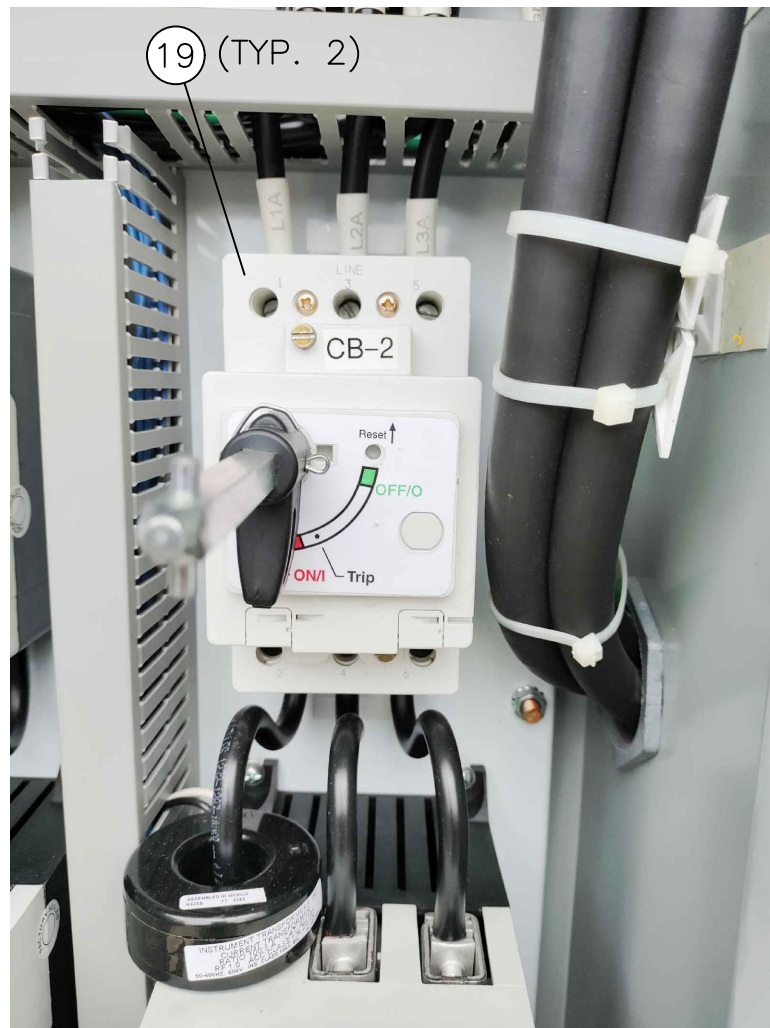
MOTOR CIRCUIT PROTECTOR DETAIL
