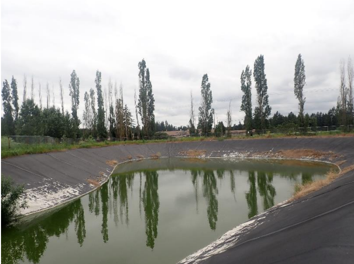
Photo 3. Large concrete settling pond
