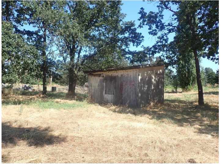
Photo 2. Grass growing over compressed rock
