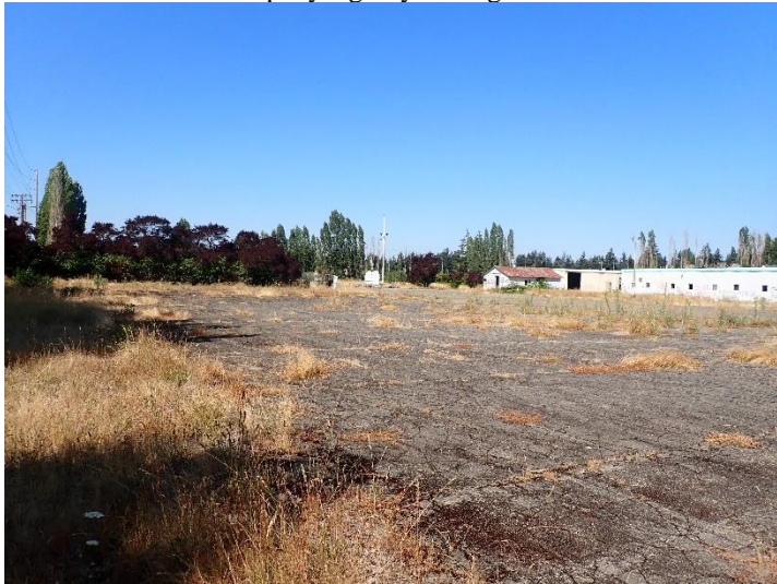
Photo 21. Large concrete parking lot on southern part of property
