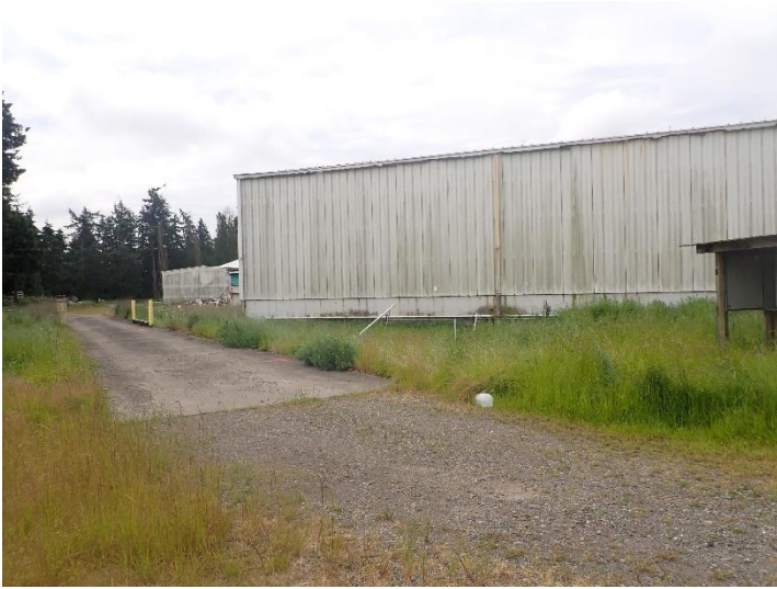
Photo 15. Internal roads and buildings
