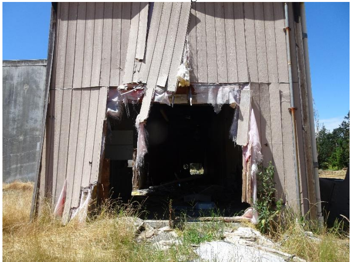
Photo 18. Partially demolished building
