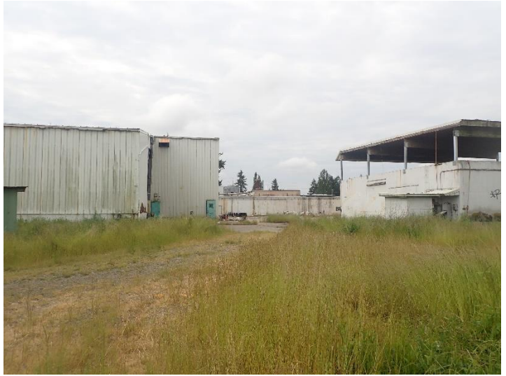
Photo 16. Internal roads and buildings
