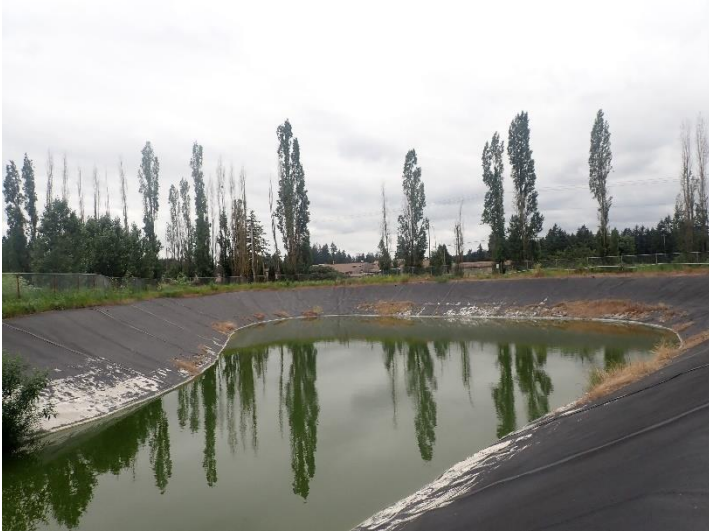
Photos 13. Settling pond
