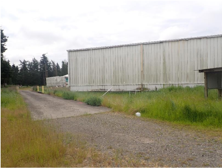
Photo 15. Internal roads and buildings
