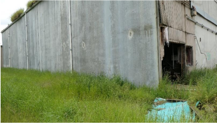
Photo 1. Abandoned building from Mushroom farm facility
