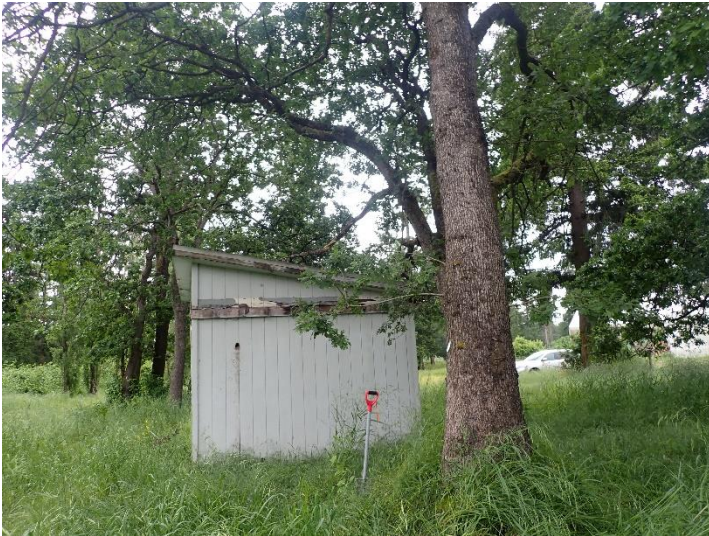
Photo 21. Existing shed adjacent to small oak stand
