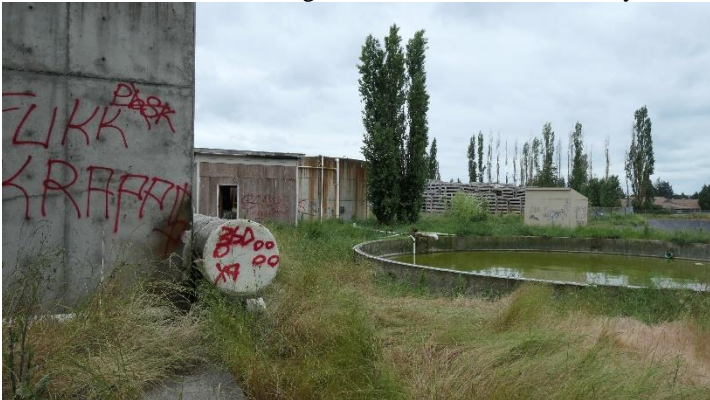
Photo 3. Abandoned buildings and derelict facility
