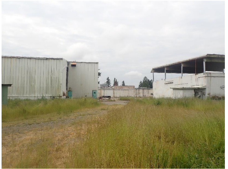
Photo 16. Internal roads and buildings
