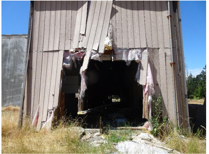
Photo 18. Partially demolished building
