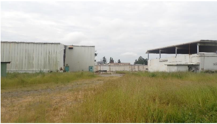
Photo 9. Internal gravel road connecting access to buildings
