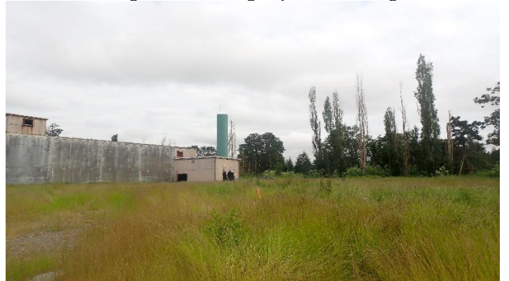
Photo 8. Compressed rock covered by grass
