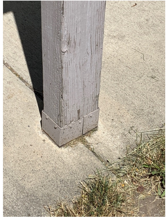
Figure 7-Post Base Bracket
