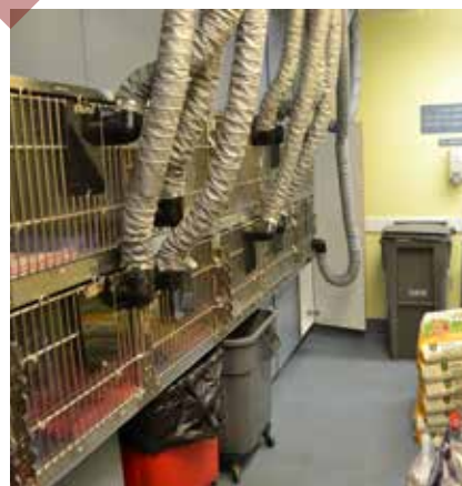
Figure 26. Ad hoc hoses are connected to kennels to provide adequate air circulation during isolation
