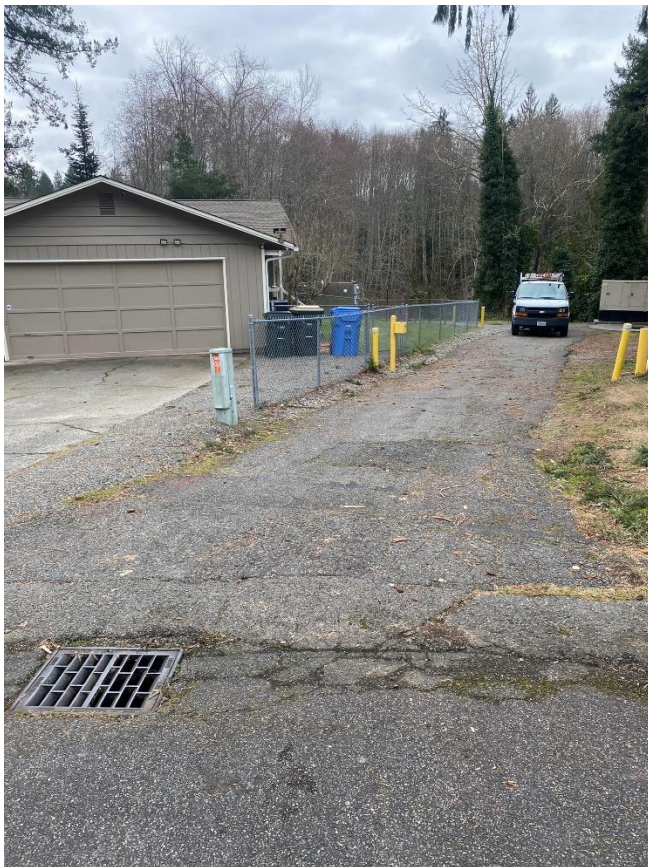
Figure 1: Existing property fence and gate
