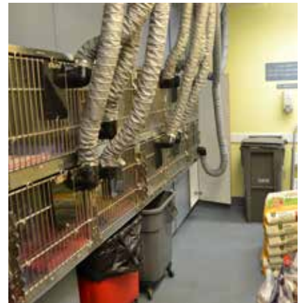
Figure 27. Ad hoc hoses are connected to kennels to provide adequate air circulation during isolation
