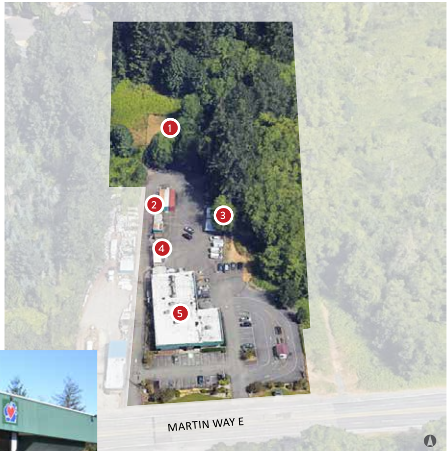
Figure 24. Animal Services facility
