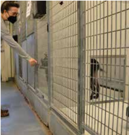
Figure 31. Divider between kennels is removed to provide space aligned with industry standards
