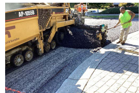
Laying asphalt in the roundabout at Rainier Rd and Balustrade Blvd in 2023
