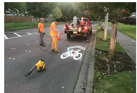
Applying shared lane thermoplastic bicycle symbols
