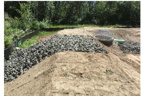
Construction of new flow control structure and emergency overflow spillway as part of modifying the existing detention storm pond at Hawks Prairie Reservoir
