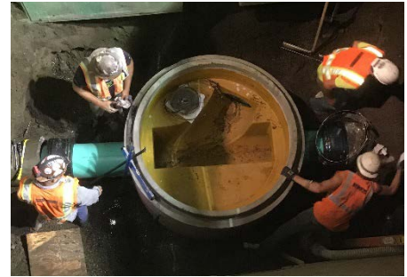
Installing a new sewer manhole as part of the wastewater replacement on Golf Club Rd
