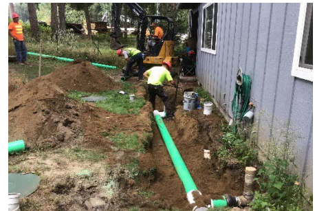
New sewer lateral installation and house infrastructure reconnection at Capitol City Golf Course
