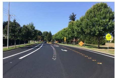
Newly installed road striping with raised pavement markers and thermoplastic lane lines along Rainier Rd in 2023
