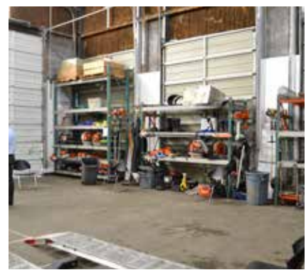
Figure 17. Parks shop is aging and functions poorly
