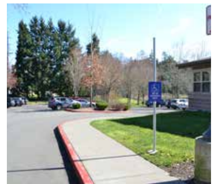
Figure 59. Parking lot slopes down and away from the Senior Center
