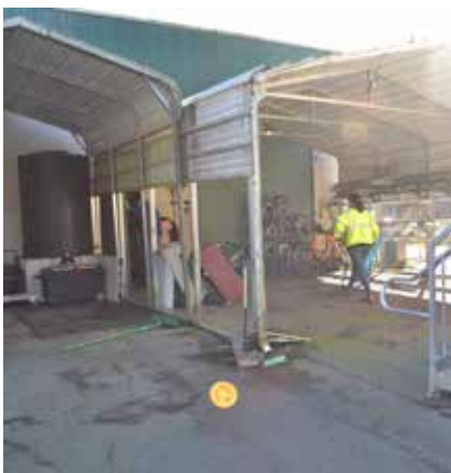
Figure 32. Open and unsecured sally port
