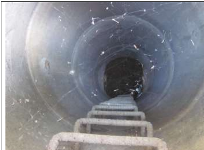
Existing structure access
