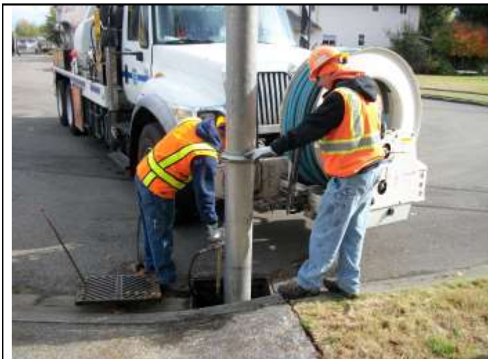
Catch basin cleaning
