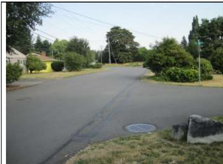
Neighborhood lacks stormwater drainage
