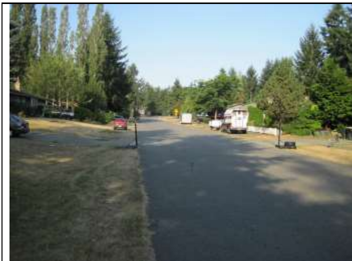
Site of future shoulder improvements, looking west.
