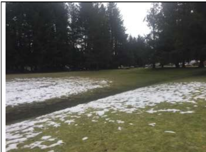
Evidence of ponding in low spots
