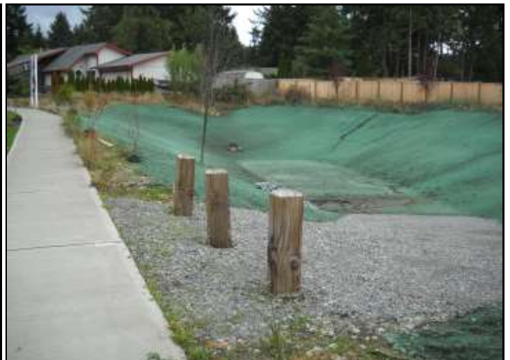
Facility under construction
