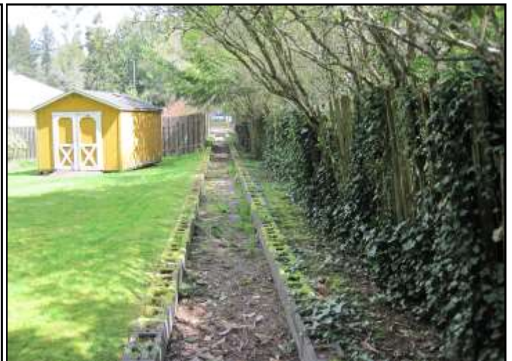
Existing above-ground overflow from facility.
