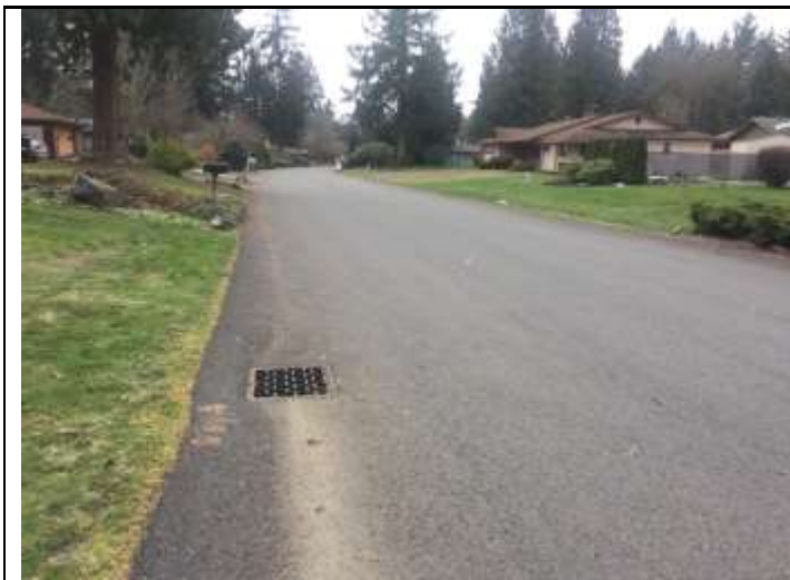
Completed Brentwood project nearby
