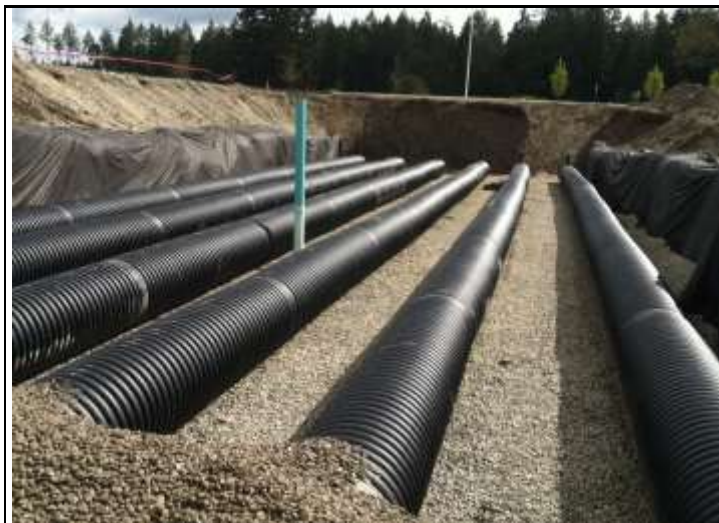
Infiltration gallery construction
