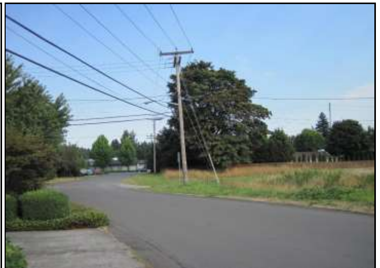
Neighborhood lacks stormwater drainage
