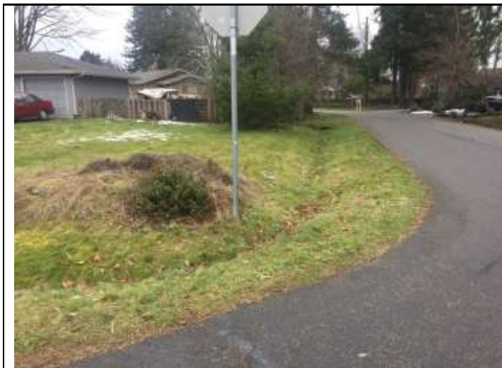
Corner with thrust block preventing conveyance through existing ditch
