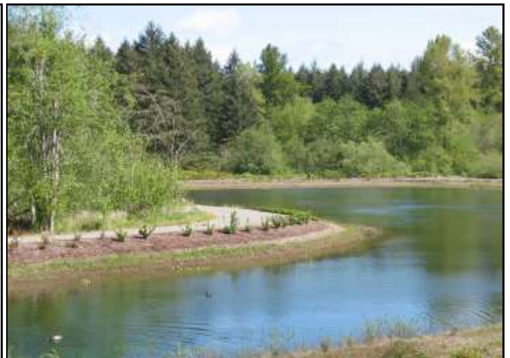
Stormwater treatment facility
