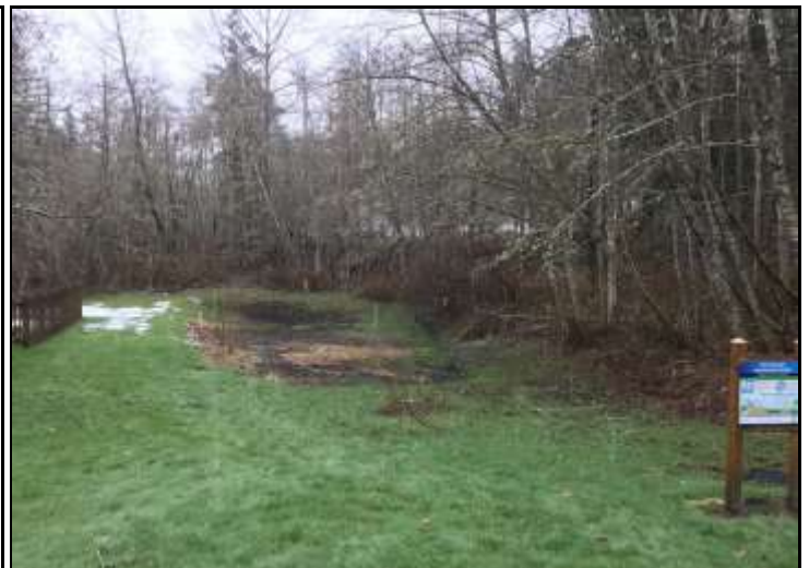
Existing stormwater pond, looking south
