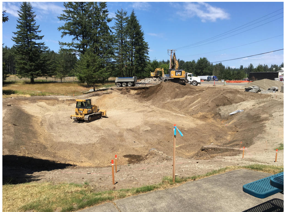
HOGUM BAY POND EXCAVATION
