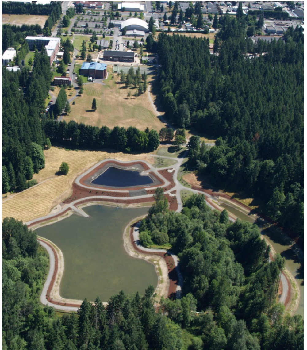
COLLEGE STORM FACILITY AERIAL
