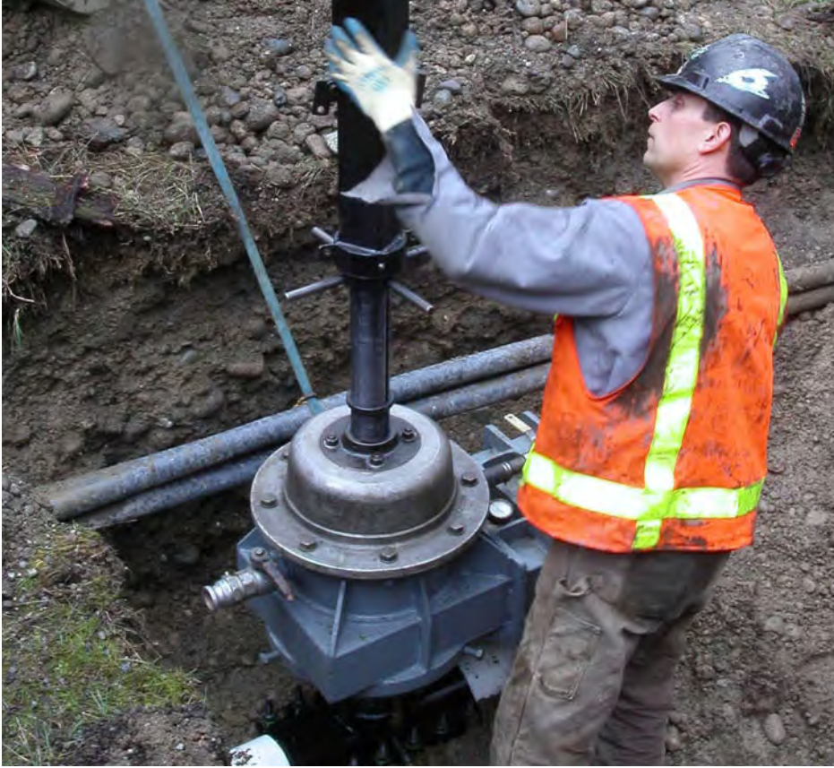
Contractor tapping one of Lacey's water lines.
