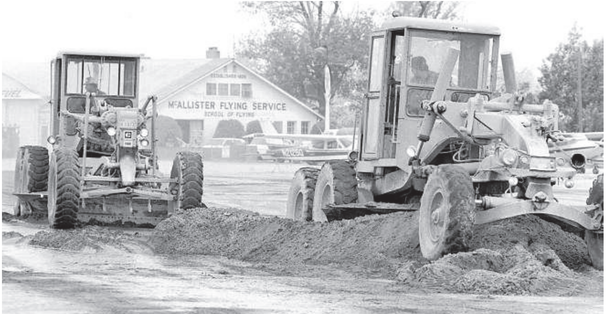
Removal of ash from Mount Saint Helens near the Yakima Airport. Photo courtesy of the Yakima Herald
