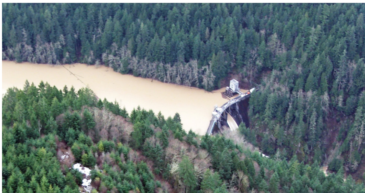
LaGrande Dam. Photo courtesy Washington State Department of Transportation
