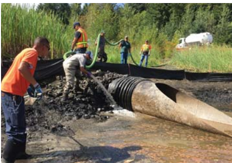
Maintenance Crews at College Regional Stormwater Facility
